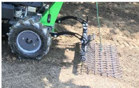
Finishing raking and harrowing
